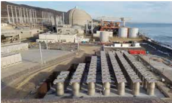
San Onofre Nuclear Generation Station (미국 캘리포니아 San Diego county)
