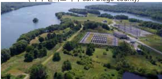
Maine Yankee Nuclear Power (미국 Maine주 Wiscasset)
